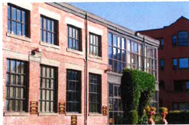
The horizontal articulation of the building is emphasized with the window patterns
