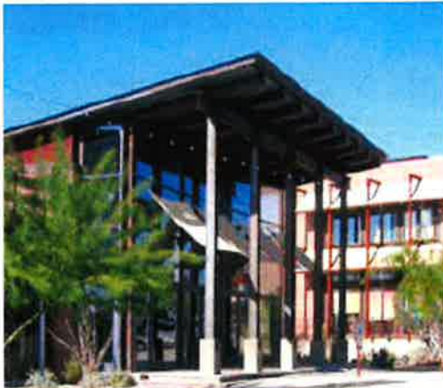
Entry awning provides shade and covered seating area
