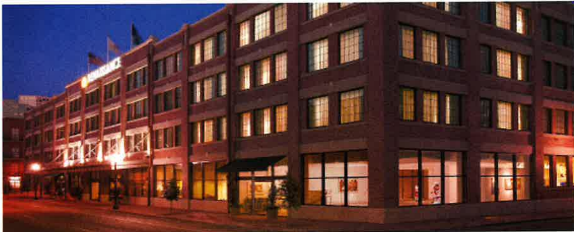
Large glazed openings allow in plenty of natural light to improve the well-being of workers.
