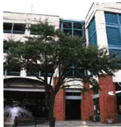
Central lobby spaces to access garage
