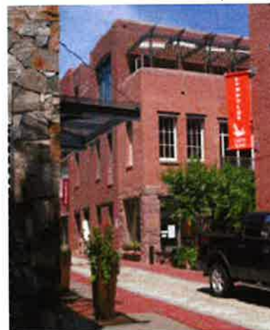
Habitable outdoor space and roof pergola with architectural detailing
