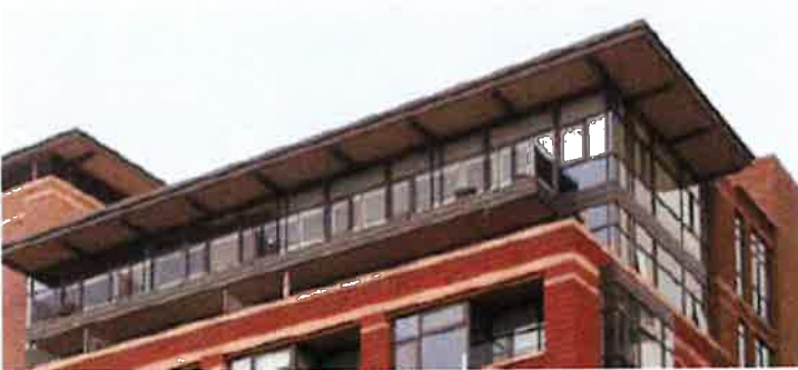
A projecting overhang as the roof form for a larger mixed-use building
