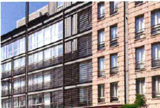
Window placement of punched openings and skeletal systems
