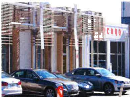
Shading and screening devices improve indoor environment and add architectural interest
