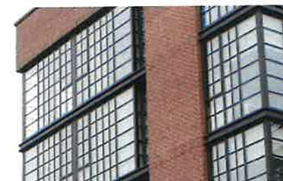
Glass curtain wall
