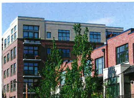
Transition from brick to stucco on upper stories
