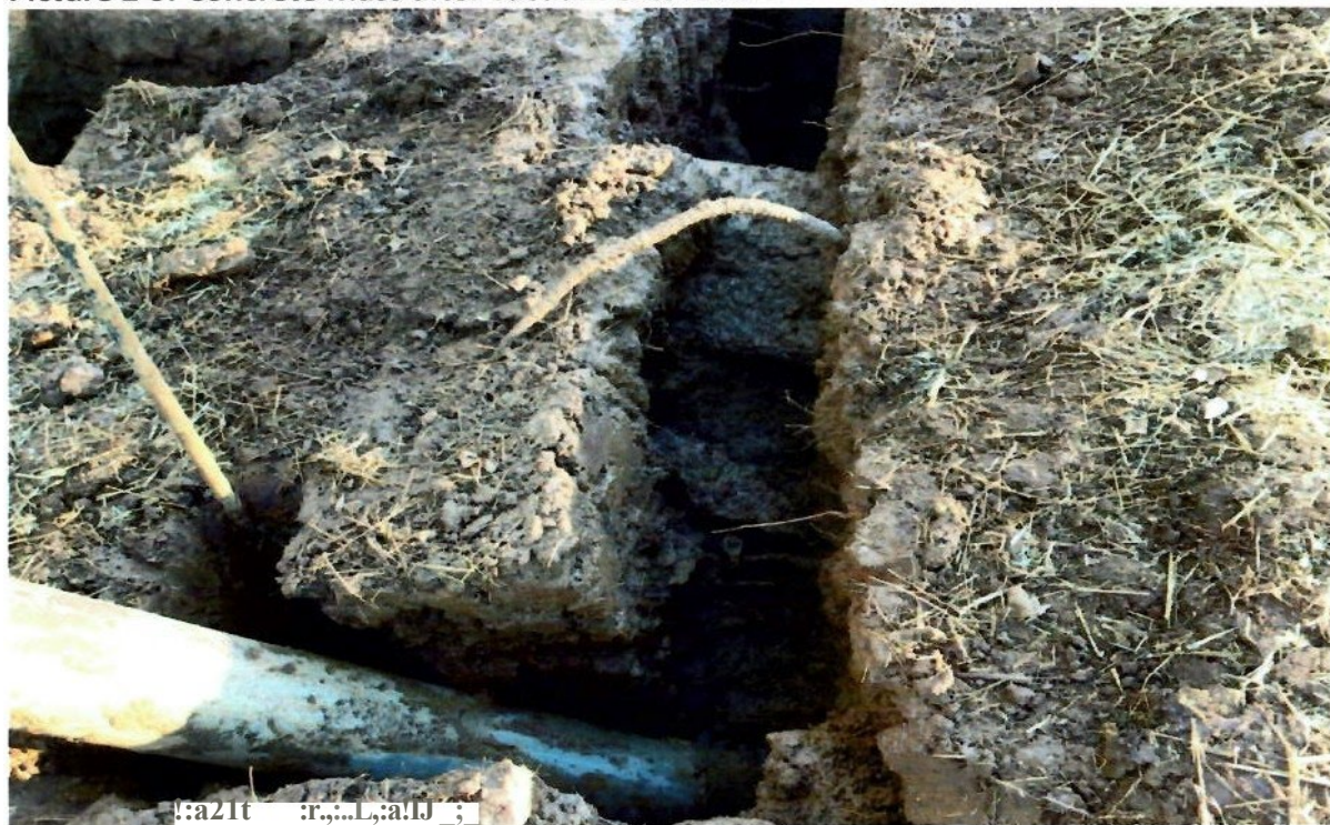
Picture 3 of Concrete Mass after vacuum excavation:
