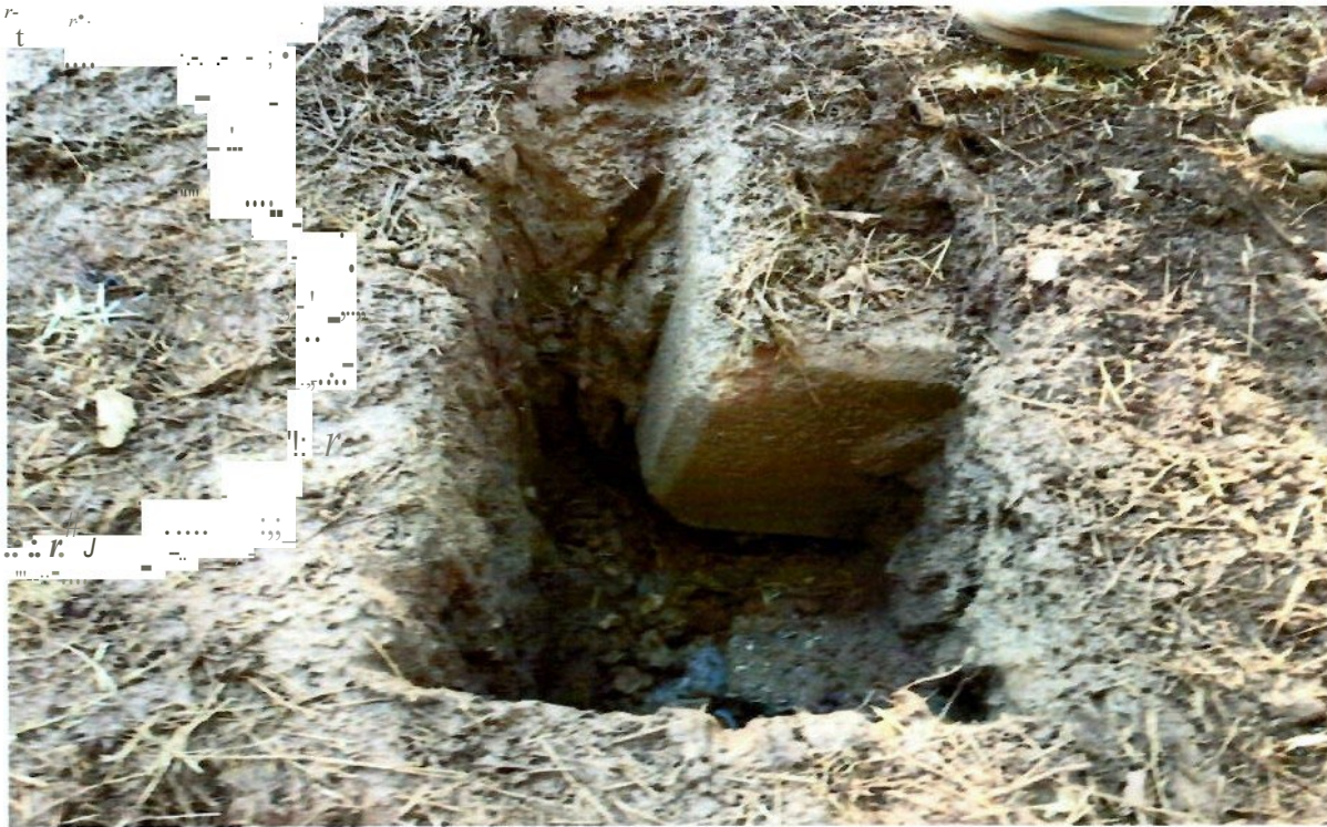
Picture 2 of Concrete Mass after vacuum excavation:
