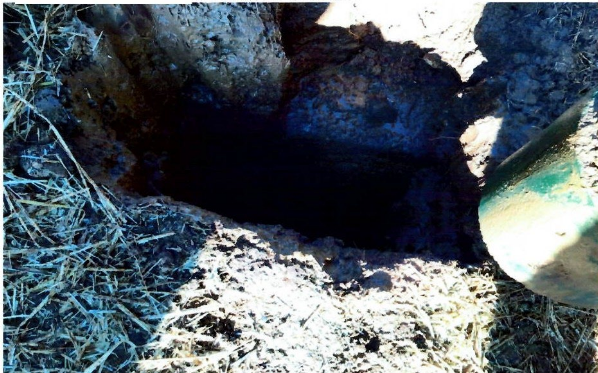
Picture 4 of Concrete Mass after vacuum excavation:
