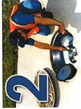
Tighten center bolt to secure pan in place
