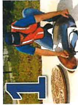
Position LockDown pan into manhole
